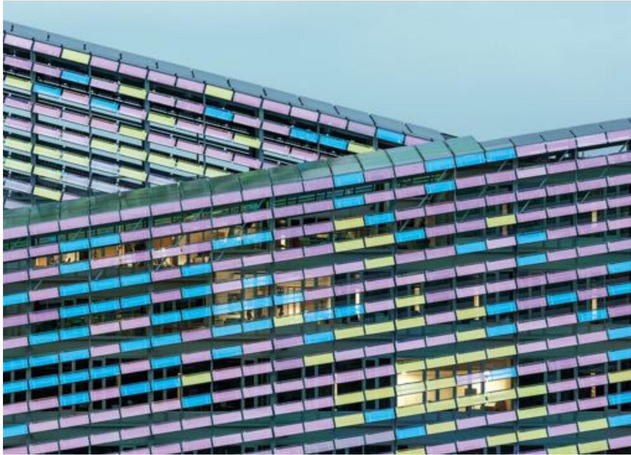
The scale-like panels on the facade of Métropole Rouen Normandie are coated with a layer of metal oxide, which gives them a colourful, iridescent appearance
