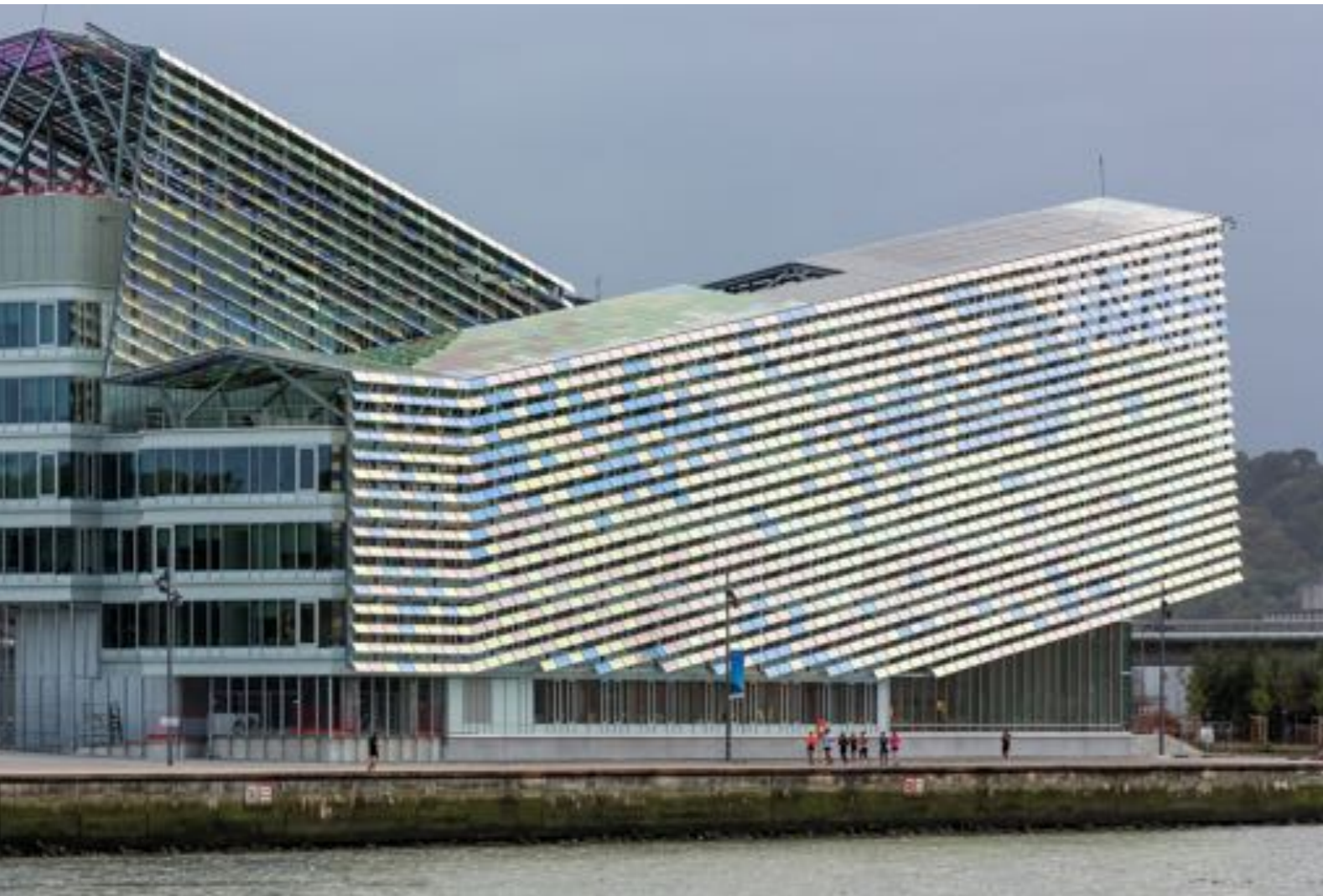
Reminiscent of the works of the French impressionists, in particular Claude Monet, the building's innovative skin reflects the light from the surface of the river below, and the changing Normandy sky
